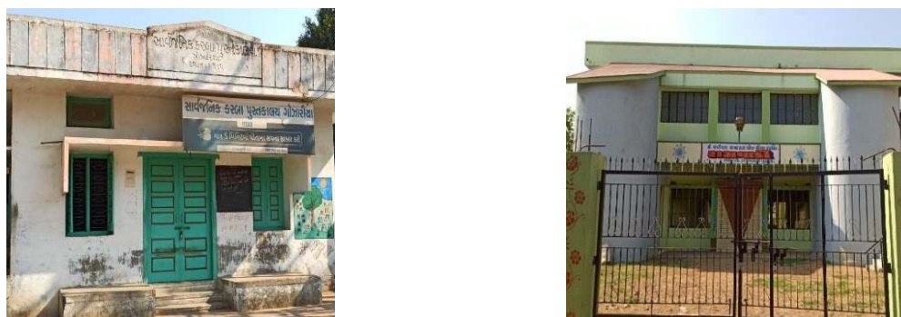
Figure 7 Library and Community Hall
